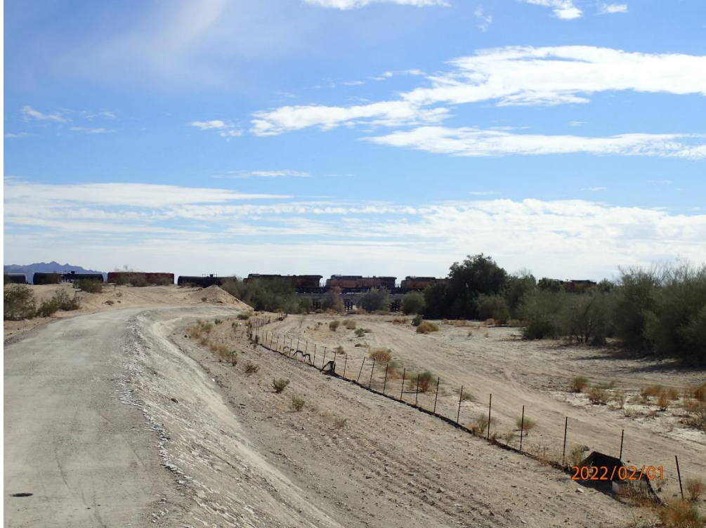
13. Southeasterly from the highway to the U.P.R.R. trestle across Fortuna Wash.
