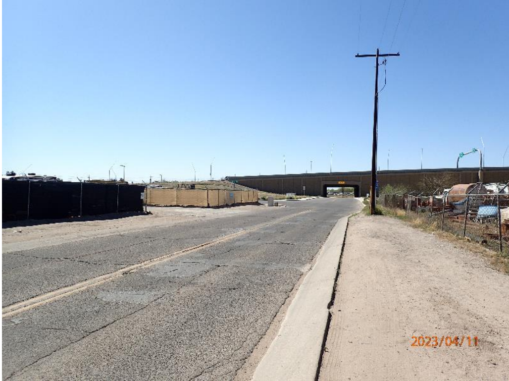
Looking south on Davis Avenue, subject property to the right.
