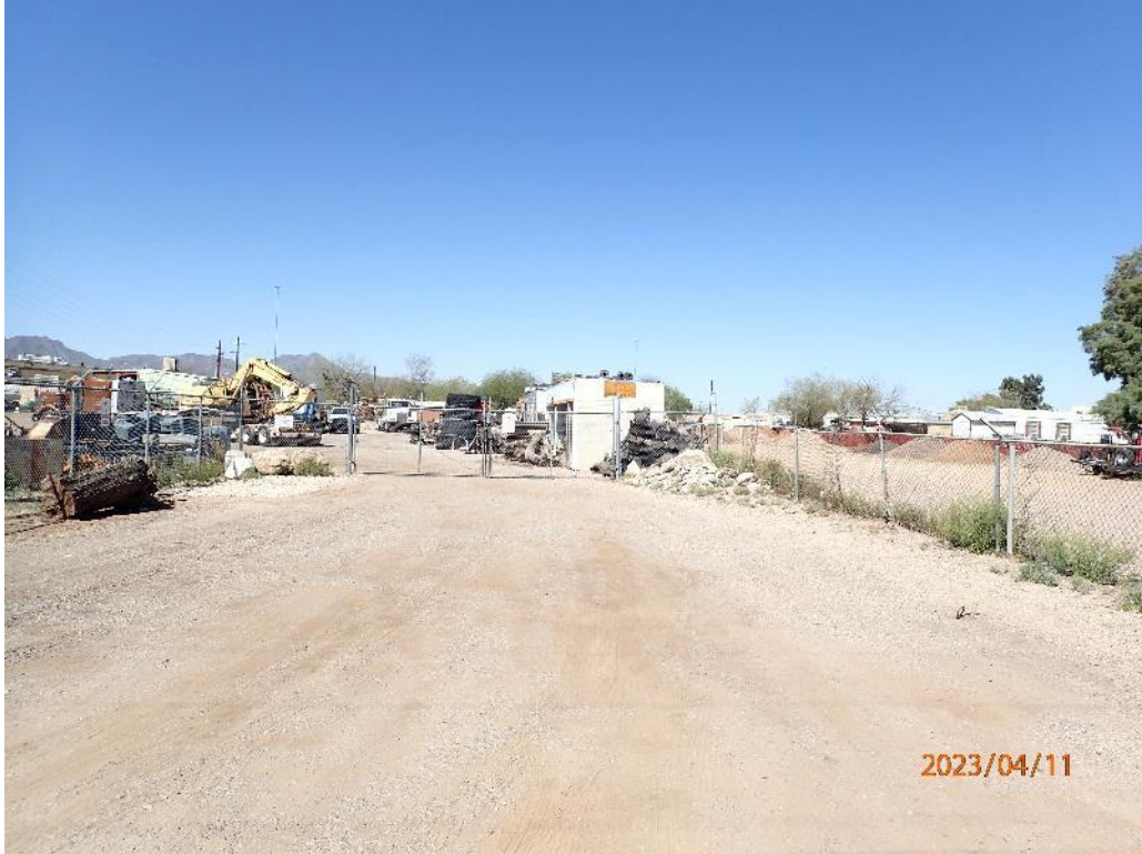
Looking west across northern portion of the subject property from Davis Avenue.
