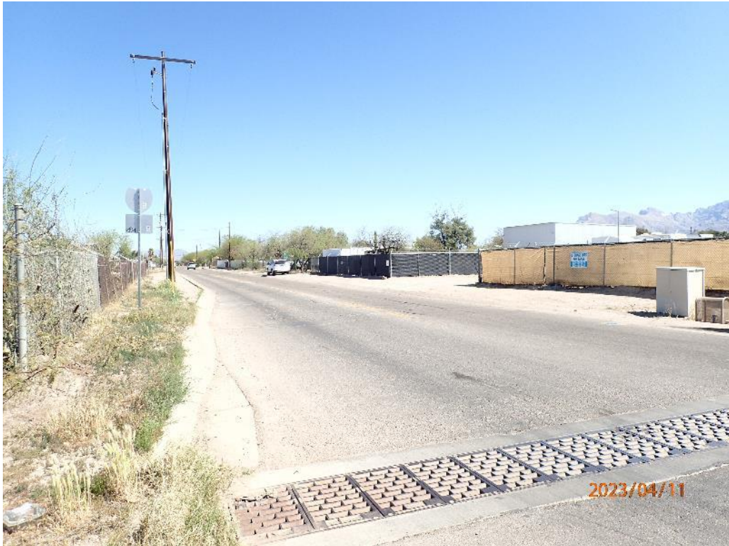
Looking north on Davis Avenue, subject property to the left.
