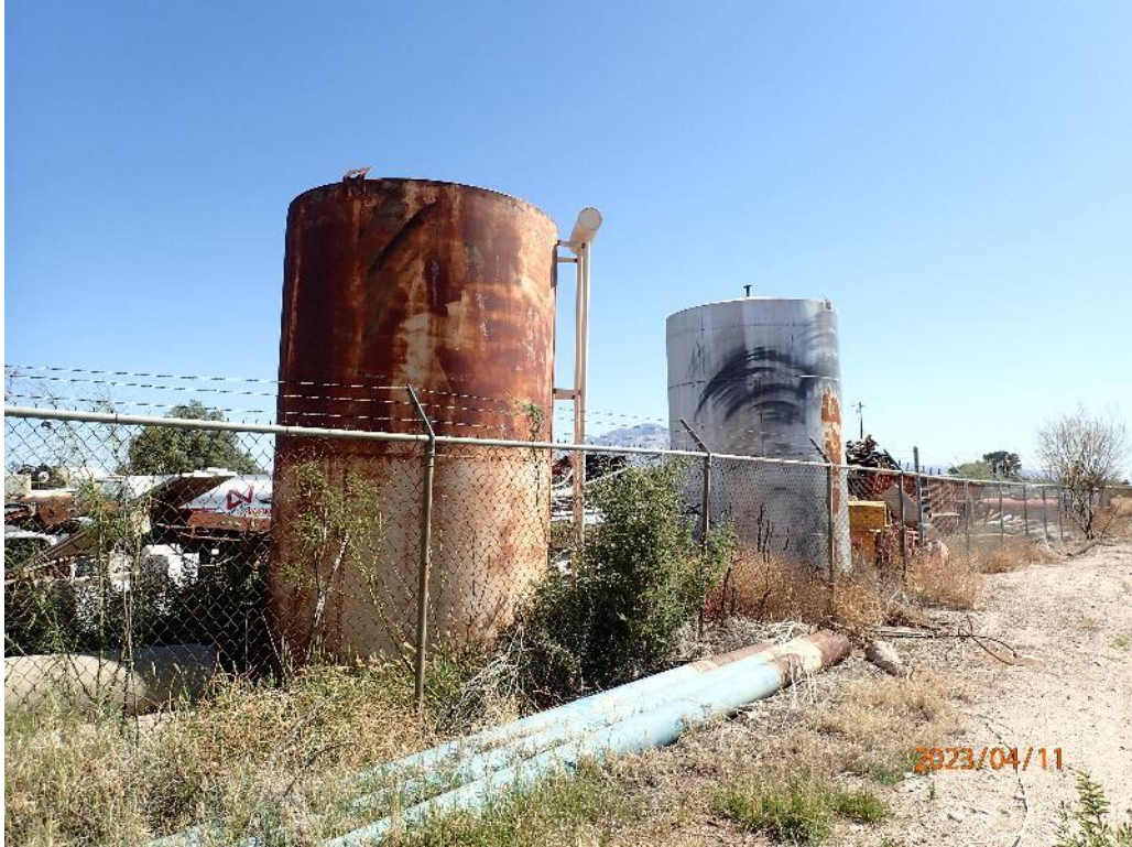
View along south boundary of the subject property.
