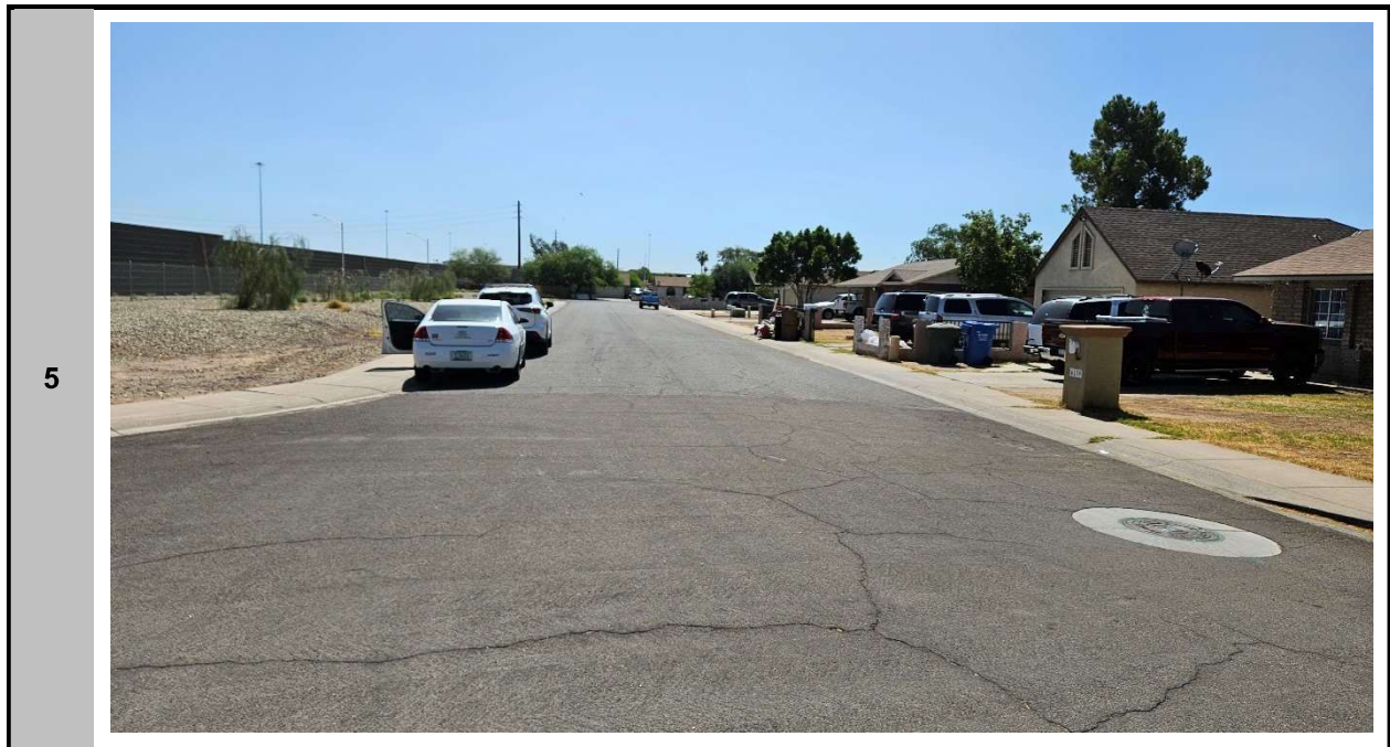
View east along Belleview Street at 62 nd Avenue
