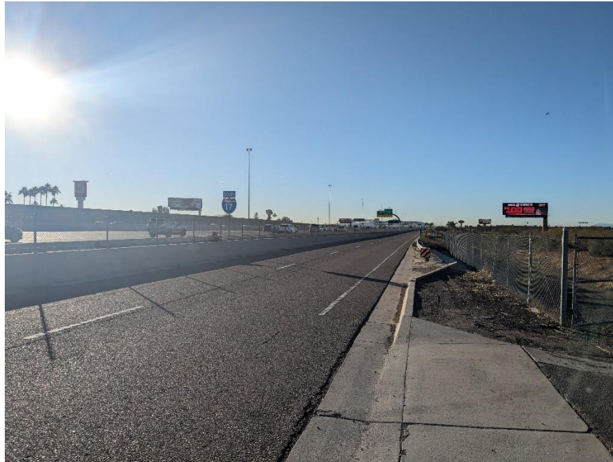
I-17/Black Canyon Hwy (frontage road) looking south from 27 th Av (155203495)
