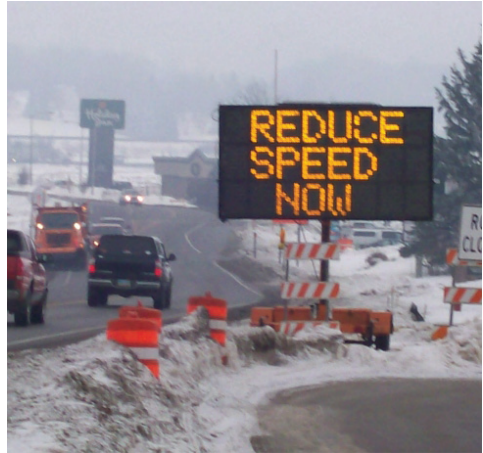
Example shows a reduced advisory speed limit due to sharp curve with either a substandard clear zone or inadequate buffer zone for errant vehicles.
