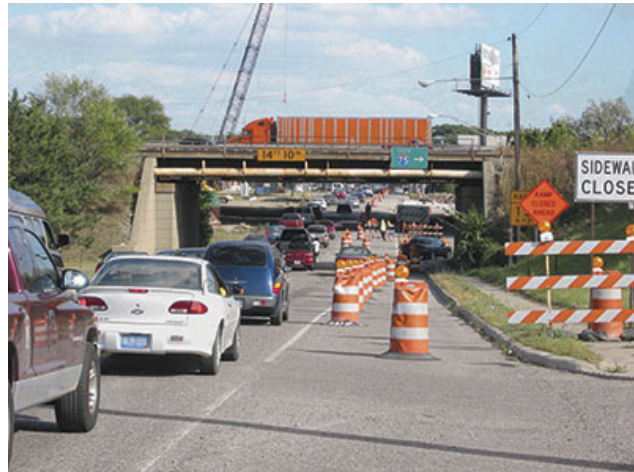
Figure 1: Work Zone Traffic 1
